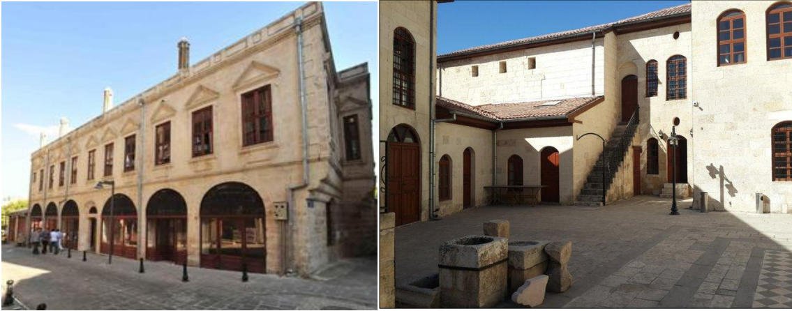
Figure 2. (a) street facade of the building,
